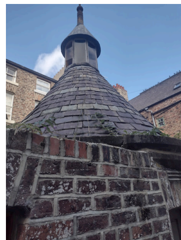
The Spa Well roof in September 2020, with weeds in guttering, damage to the cupola, and loose tiles (photo by Fiona Clewlow)
